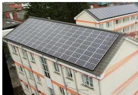
Figure 3. Solar PV added to roof.
