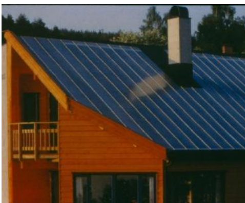
Figure 2. Integrated Solar PV roof
