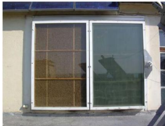
Figure 6. Integrated PV window screen.
