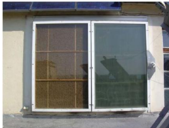
Figure 6. Integrated PV window screen.
