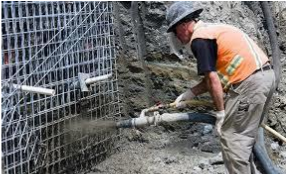
Figure 1. Protection of surface of vertical or inclined rocks. Source: http://www.belpacific.com/services/shoring-foundation-services/wet-dry-shotcrete ; accessed 15.04.2016.
