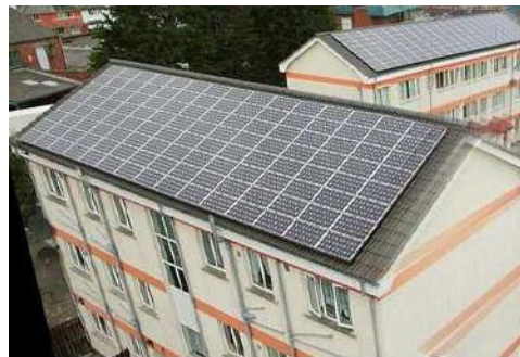
Figure 3. Solar PV added to roof.
